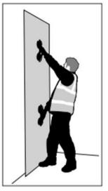
Ensure the bottom edge is correctly in place then push the panel back firm against the wall and apply pressure to all areas of the panel to make sure the TopSeal adhesive grabs to the wall.
